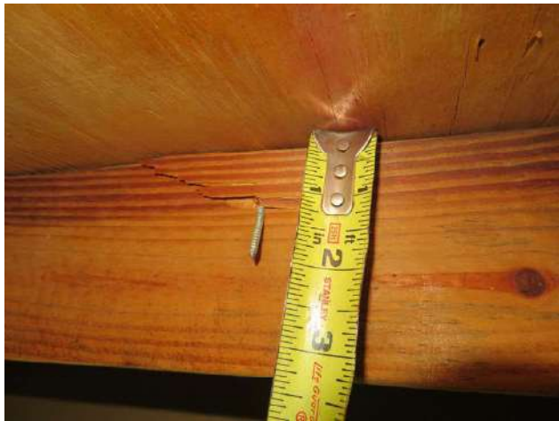
NAIL ATTACHMENT - 8D NAILS
