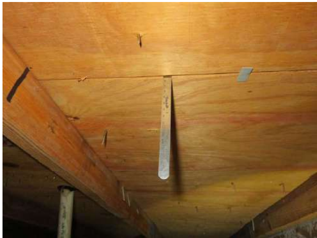
SWR - PEEL N STICK OVER ENTIRE ROOF DECK
