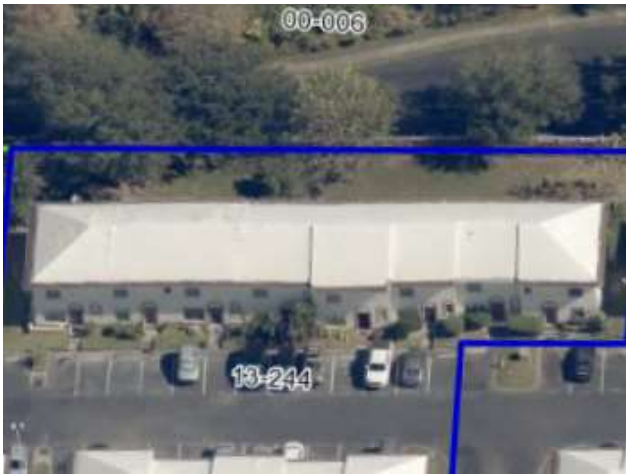
AERIAL VIEW SHOWING ALL HIP ROOF
