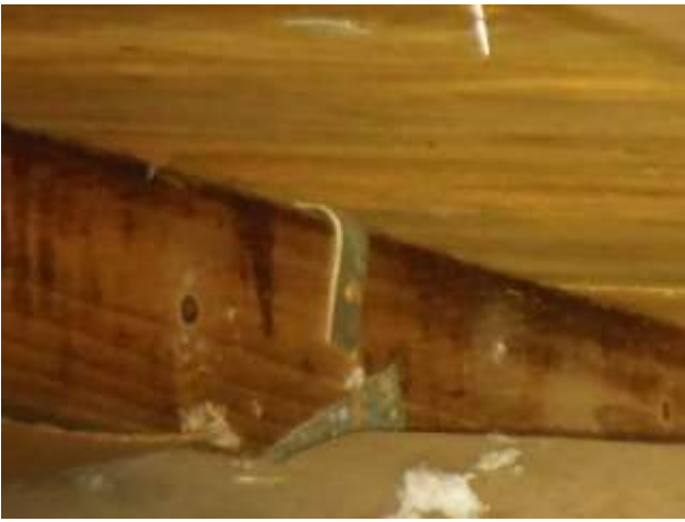
ROOF TO WALL - SINGLE WRAPS
